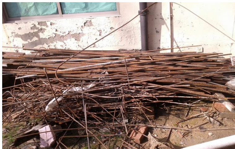
Figure 2.1 Waste of steel reinforcement
