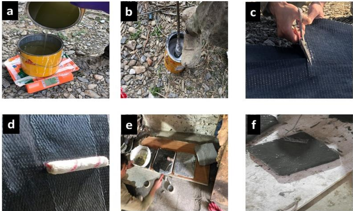
Figure 3.4:(a) Mixing of binders (b) Application of resin/ adhesive (c) Cutting of CFRP (d) Hand roller removing undulations (e) Fixing CFRP with hand roller (f) CFRP wrapped sample
