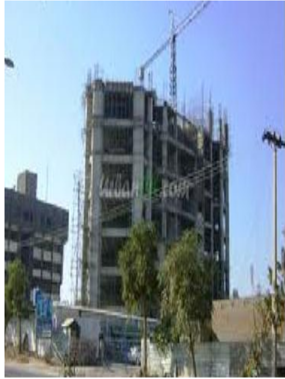
Figure 5- 3 Under construction View of OEC
