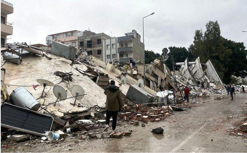
Fig 3. Earthquake in Turkey and Syria (Photo credits to BBC News)
