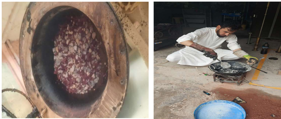
Figure 3. 14: Automatic & Manual HMA mixing
