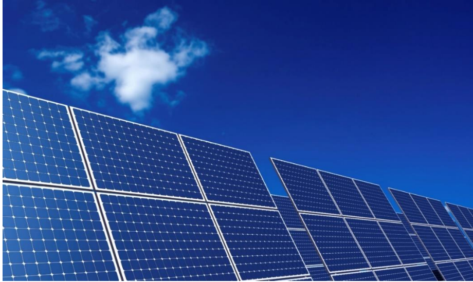
Figure 7: Solar Energy Farm
