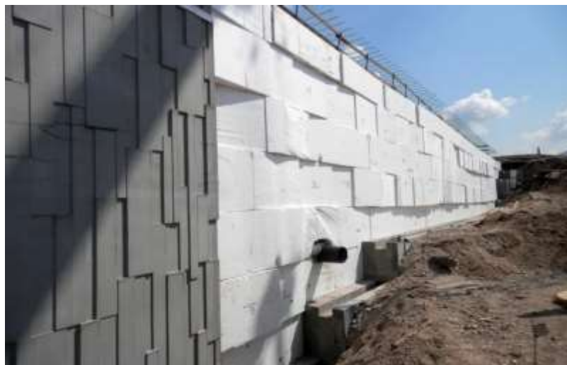
Figure 2.3 Application of Geof foam at Bridge Abutments [60]
