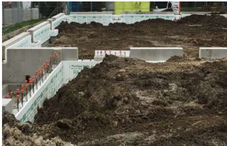
Figure 2.4 Application of Geofoam along the wall [78]
