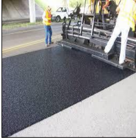
Figure 2.2. Asphaltic concrete mix (www.pavingorleans.com)
