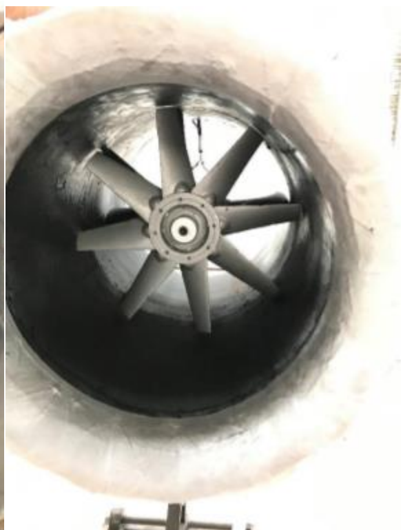
Figure 28: Engine and fan installed (b)
