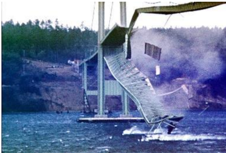
Fig 3.1-(a) Structural Failure of Tricoma Bridge in 1940
