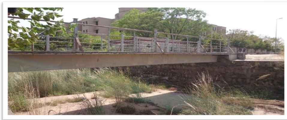
Figure 9 Picture of Selected Pedestrian Bridge
