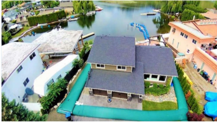
Fig 2.15: Illustrates the arrangement of water bloc barrier
