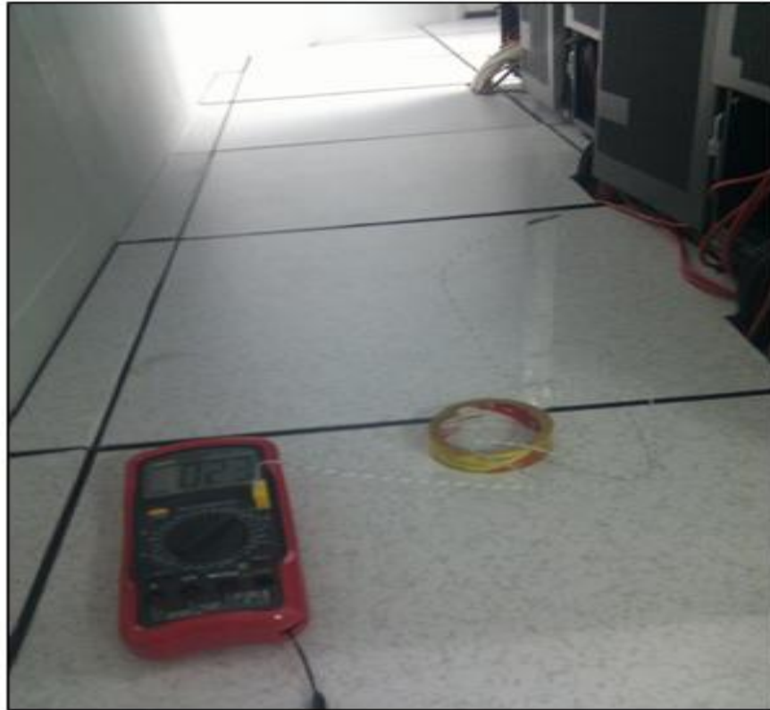
Figure 4.10: Temperature probe used for obtaining temperature data behind racks
