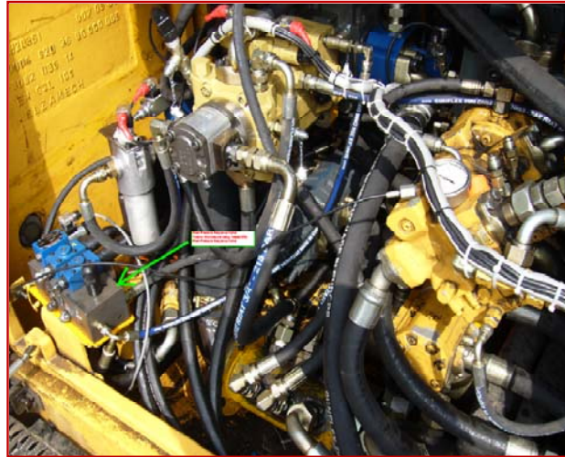
Fig 6.4: Old and New Hydraulic Circuit Valves installed in the crane LIEBHERR HS885HD with the pump for Testing Purpose.
