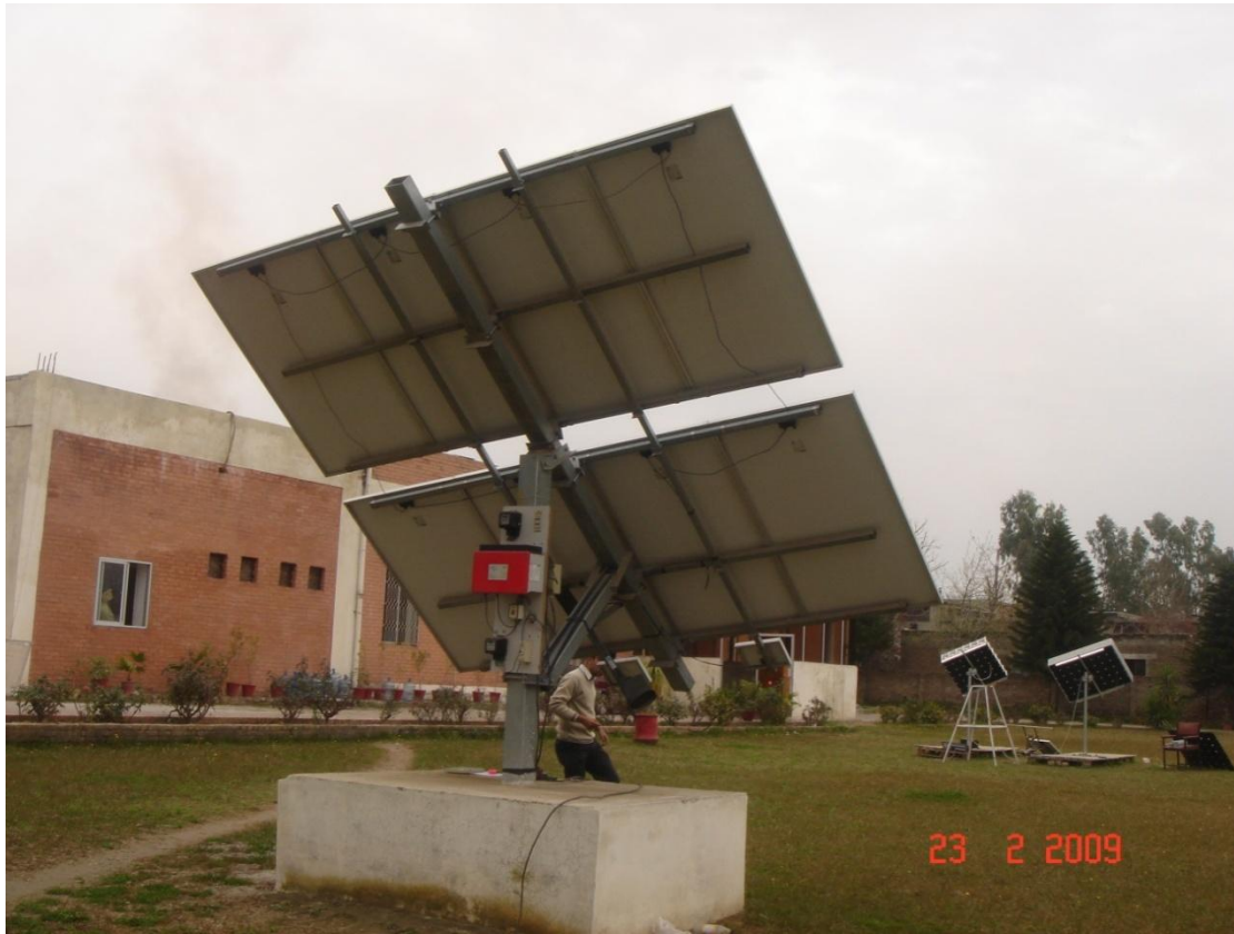
Figure18. A View of the tracking system
