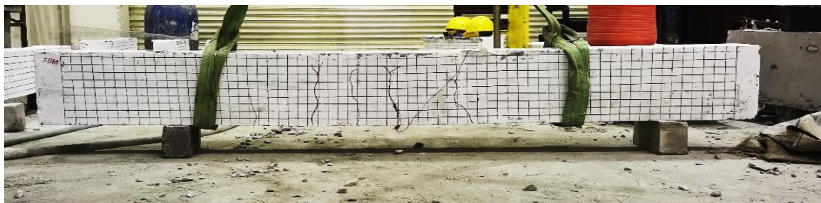
Failure pattern at Drop Height 1.7 m
