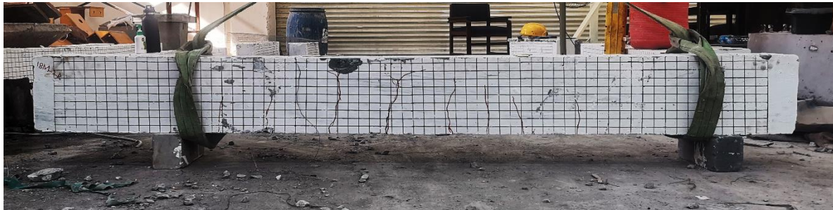
Failure pattern at Drop Height 1.2 m
