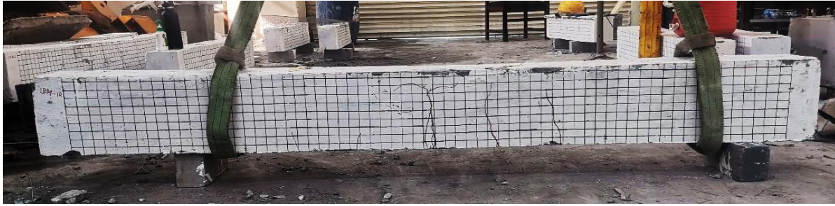
Failure pattern at Drop Height 0.7 m
