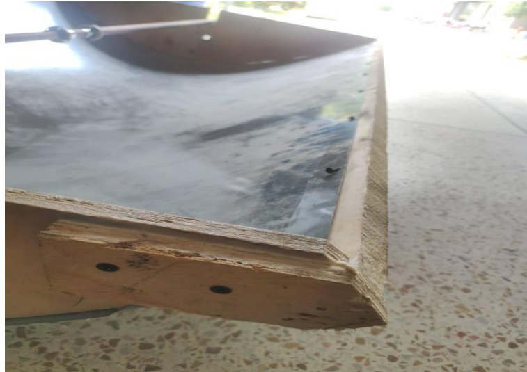
Figure 28: Wooden Supports for PSC
