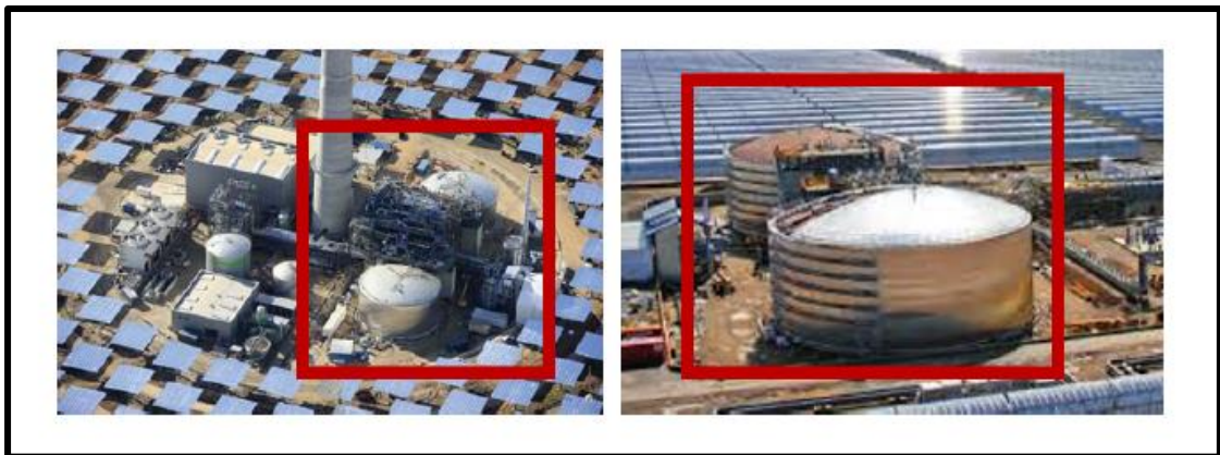
Figure 2.7: Two tanks TES systems in Gemasolar (left), and in Andasol I (right) (Source: The Andasol Solar Power Station Project - Power Technology , n.d.)
