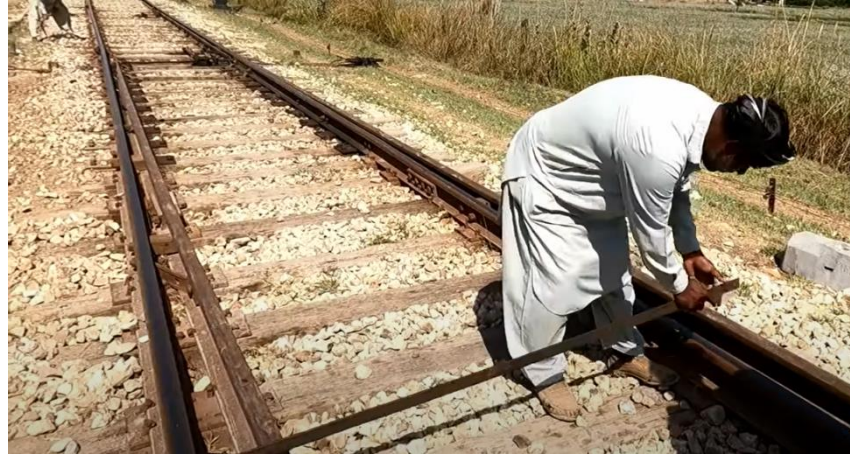
Figure 15: A railway worker measures the distance between rails near Sukkur.
