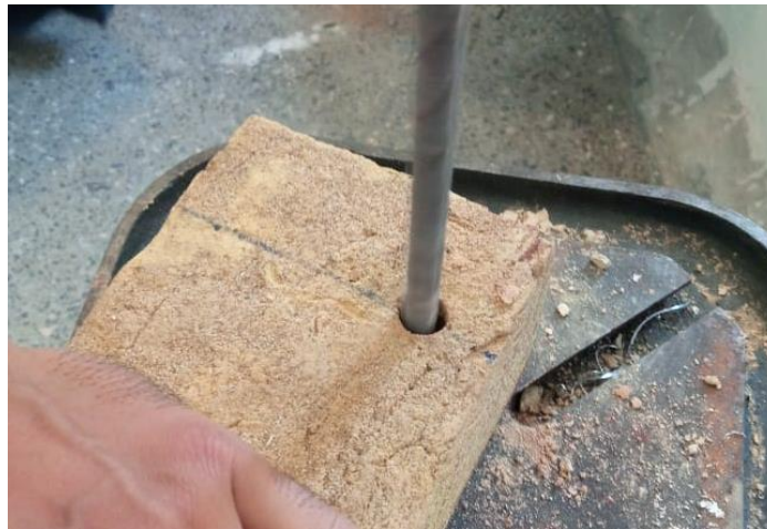
Figure 3. Drilling of Holes in Brick
