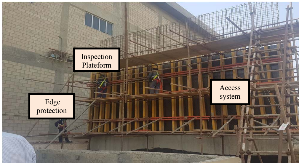
Figure 4-9- Safety Measures Adopted to Achieve Modular Formwork Benefits
