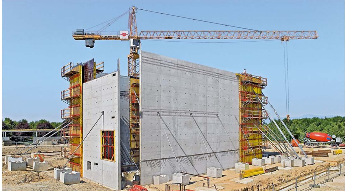
Figure 4-1- Modular Wall Formwork (50' high)
