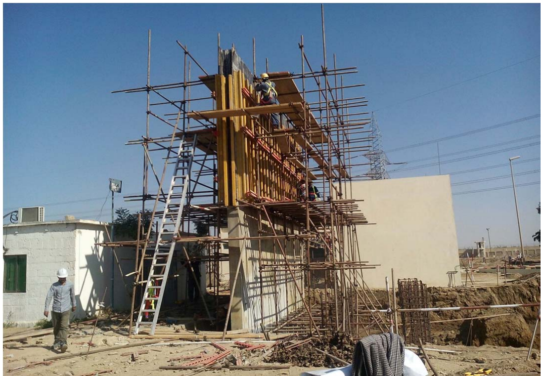
Figure 4-2 -Modular Wall Formwork (25' high)
