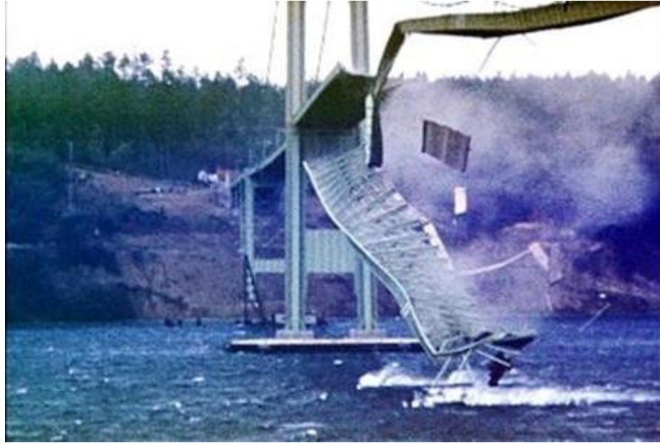
Figure 3-1: Structural failure of Tacoma bridge in 1940
