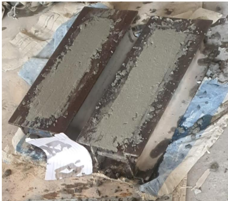
Figure 4 400mm beams casting.
