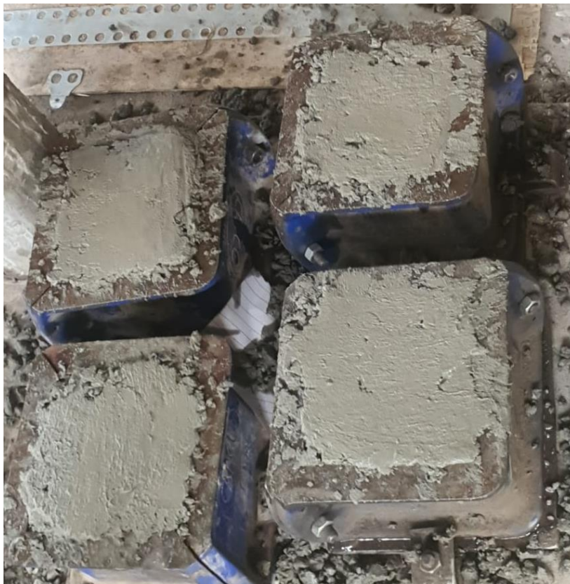
Figure 3 Cubes (150 x 150 x 150) during the casting
