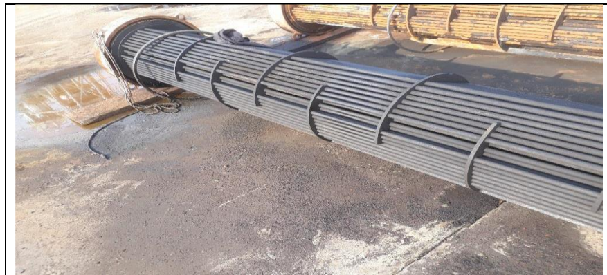
Figure 19. Flushing for removal of dirt through water jetting
