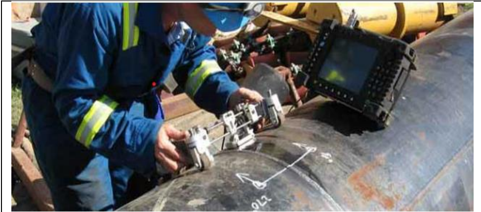
Figure 23. Application of Ultrasonic flow detection
