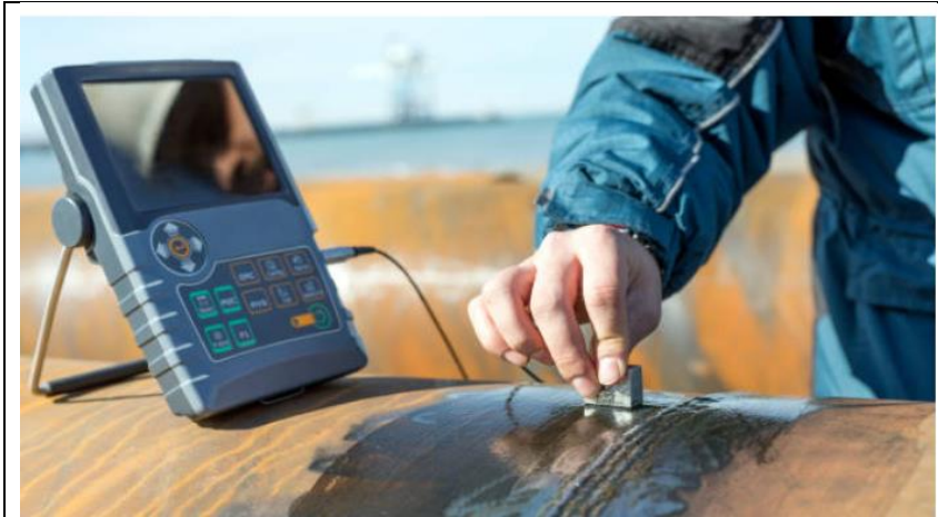
Figure 24. Application of Thickness gauging by applying gel as Couplant
