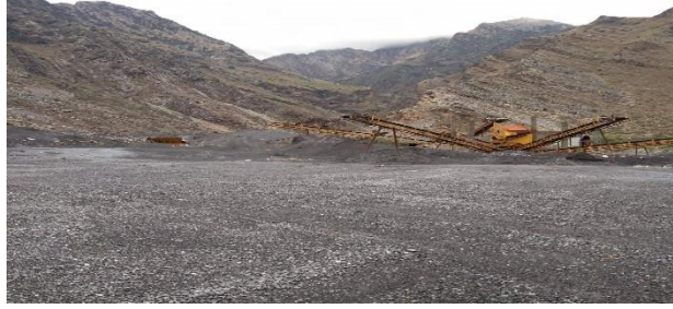
Figure 3-2 Crush Plant in Babuzai
