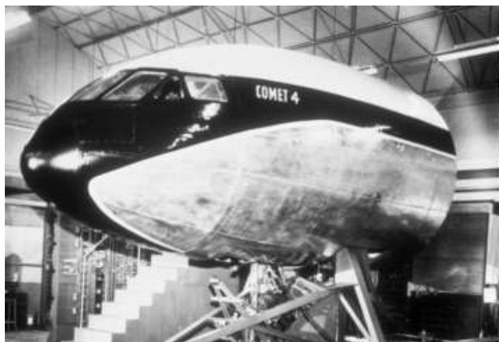
Figure 4 : First 6 DOF motion system
