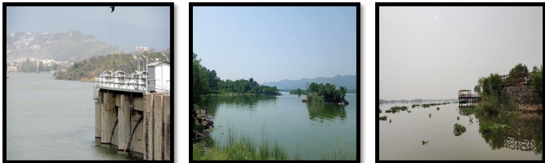
Figure 4.5 Rawal Dam observations
