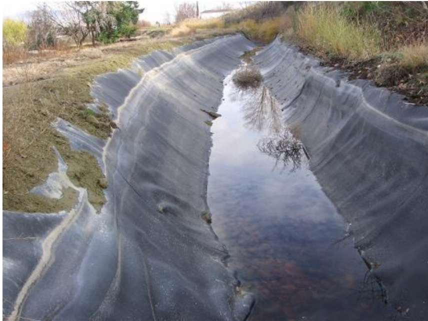
Fig 2.8 Heaving in the Lining of the channel
