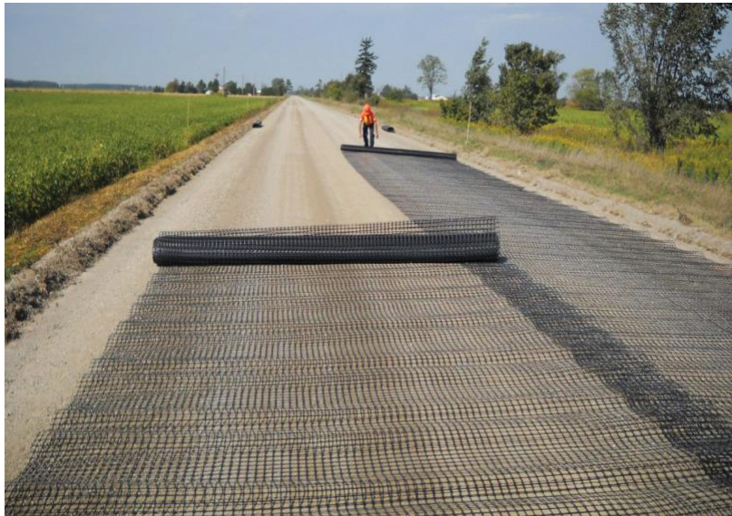
Figure 2.5: Geotextile implementation on road construction
