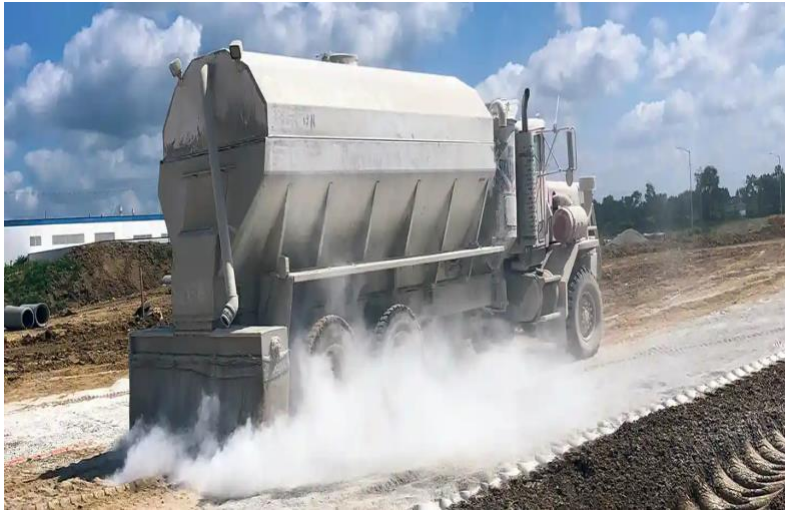
Figure 2.3: Truck spreading lime for stabilisation of soil
