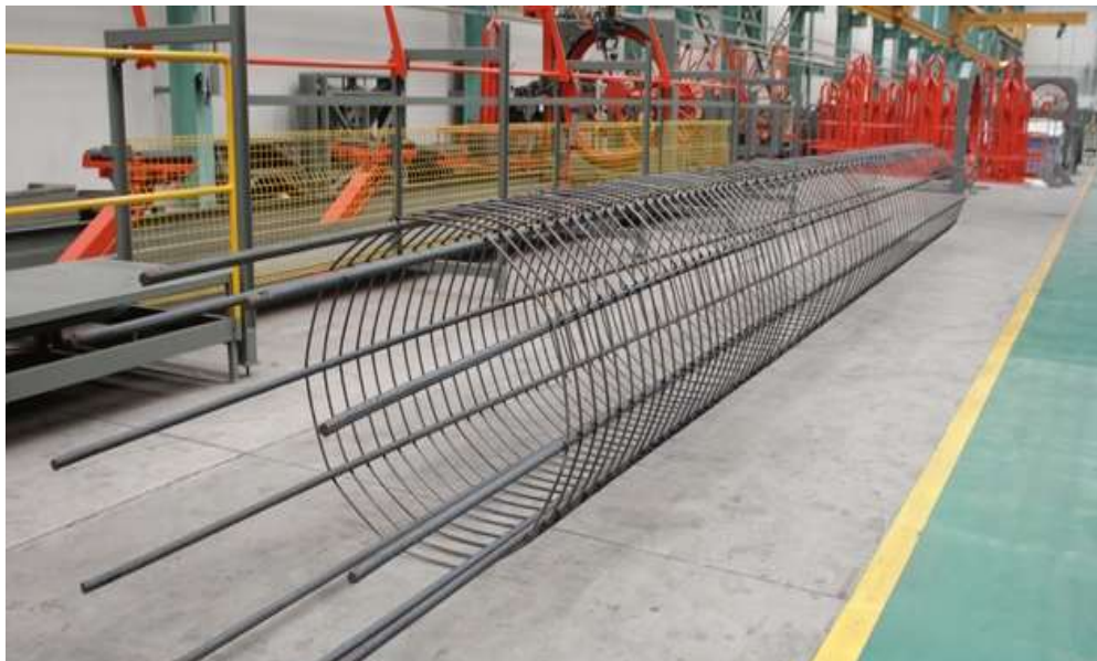
Figure 3: Pile Rebar Cage
