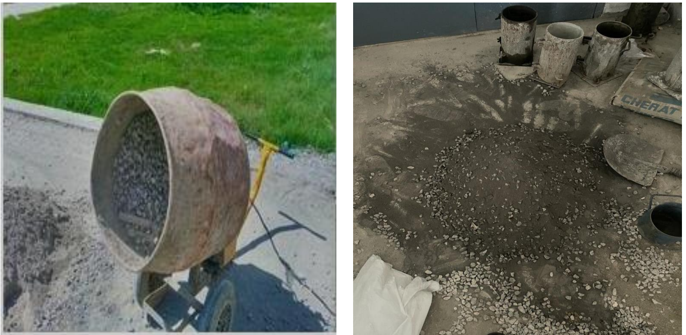
Figure 3.6 Mixing of Concrete
