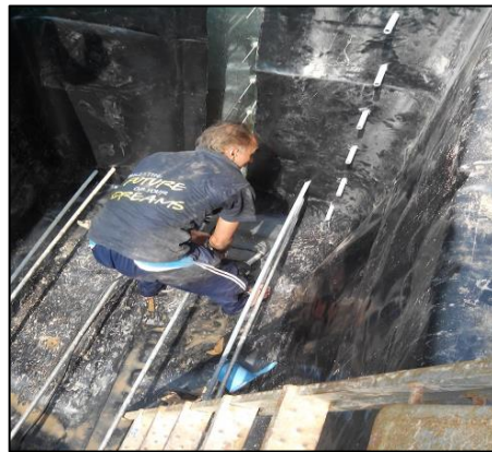
Figure 3.9: Pond lined with thickness of 1 mm High Density Polyethylene Liner
