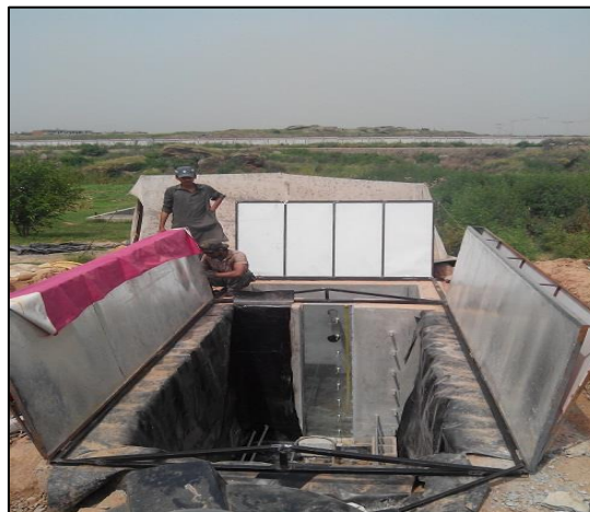
Figure 3.10: Fitting of moveable Reflectors/covers and a metal frame
