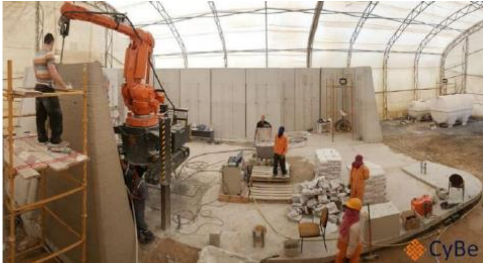
Figure 2. 14 Mobile concrete printer developed by CyBe(Teymouri 2017)
