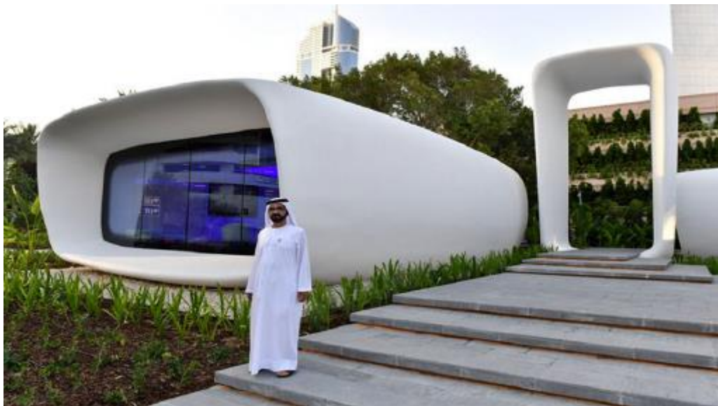
Figure 2.18 Dubai Office Building(Yin, Qu et al. 2018)
