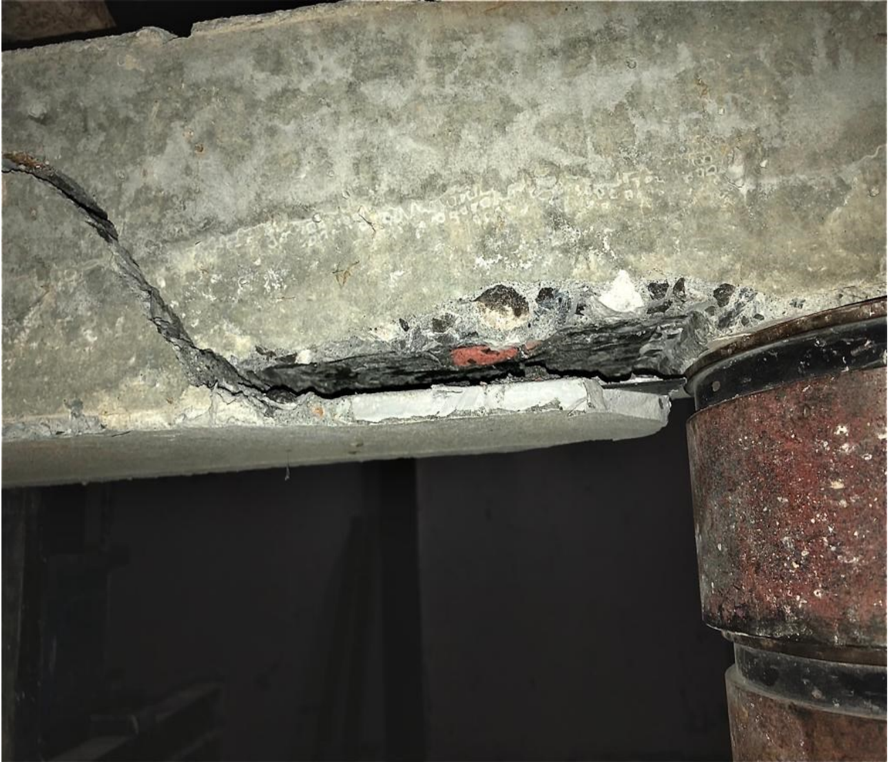
Figure 8 Experimental Failure mode of EBL (Externally bonded Laminate) strengthened beam
