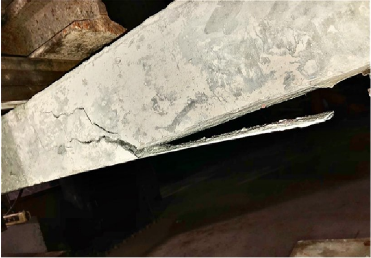
Figure 7 Experimental Failure mode of EBL (Externally bonded Laminate) strengthened beam
