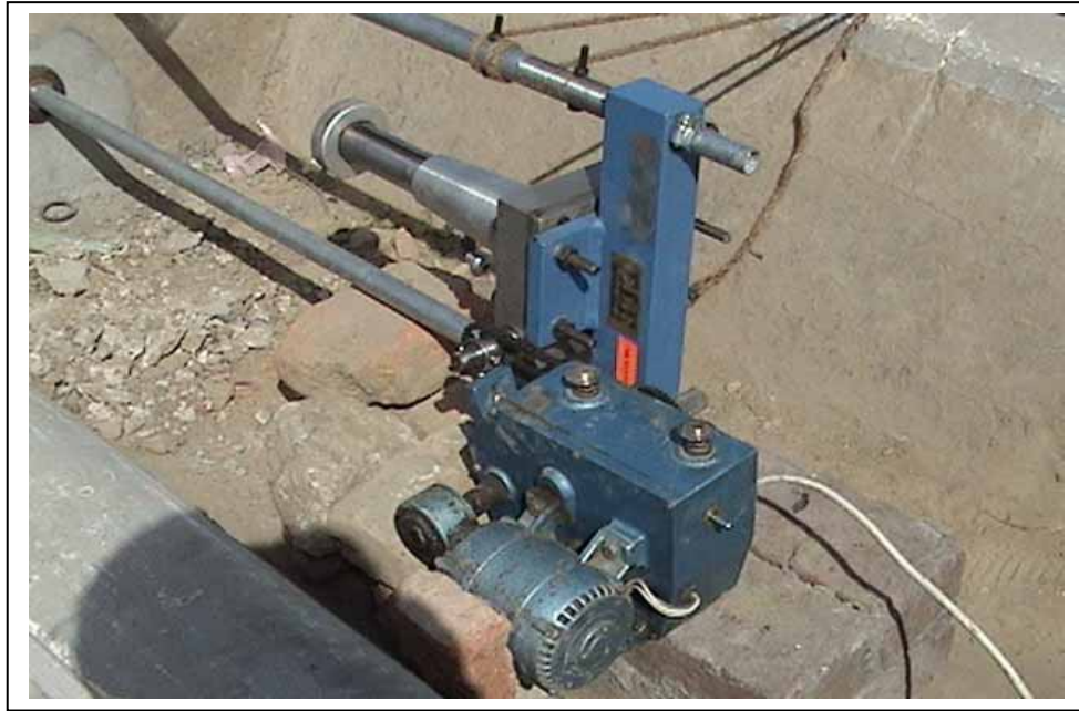
FIG.4.4. Motorized Jack for Pulling the Ropes
