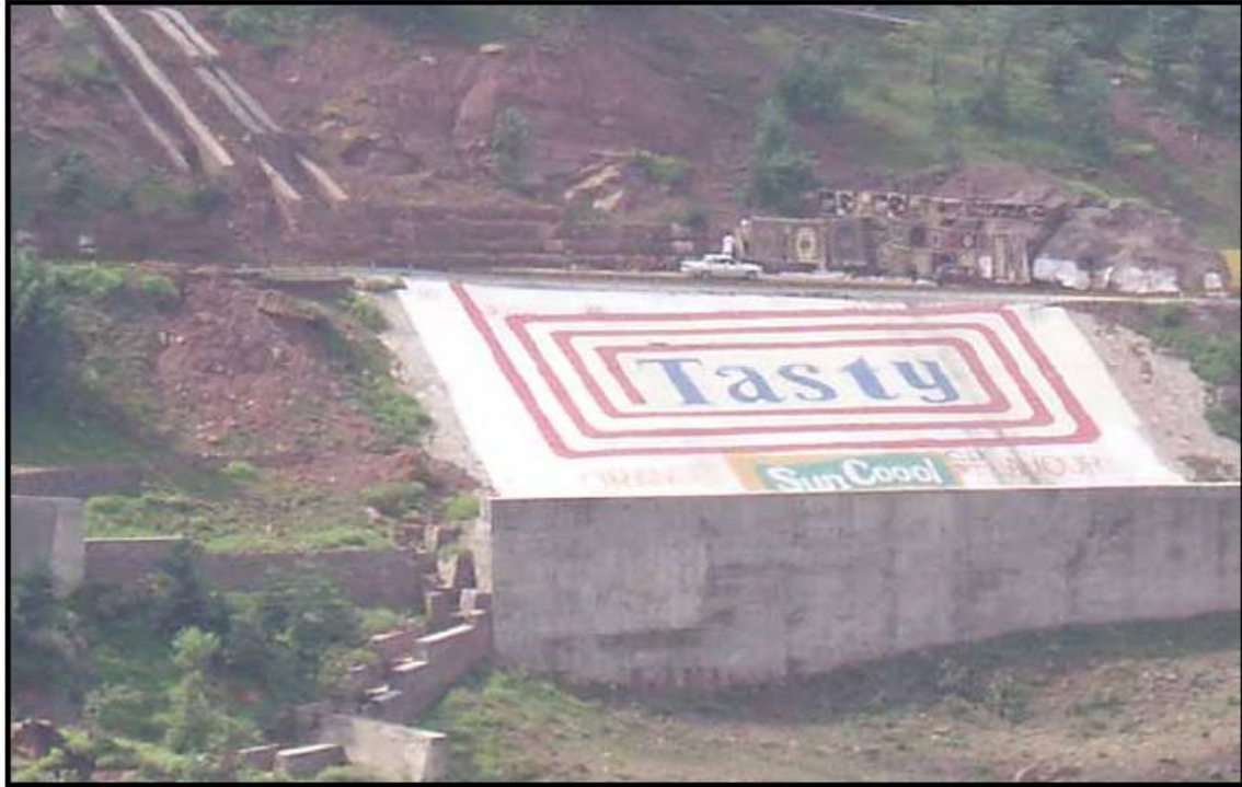
Fig. 2.5. Stabilization Work at Chitta Morr Landslide by NESPAK
