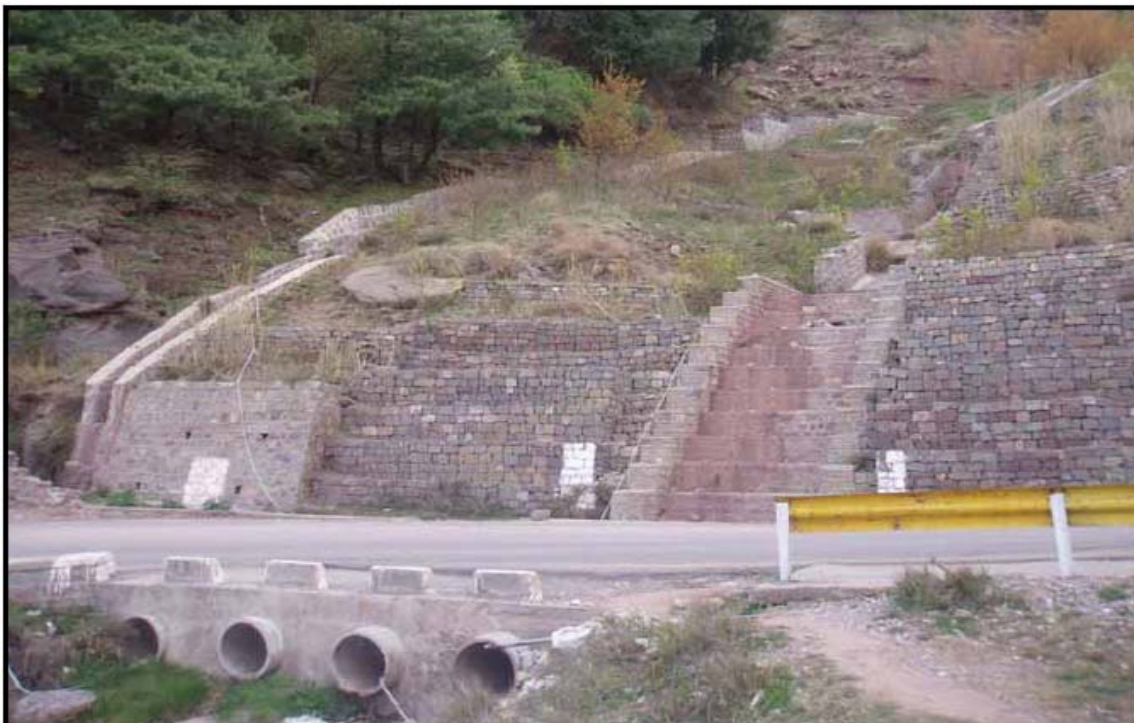
Fig. 2.6. Stabilization Work at Shawala Landslide by NESPAK
