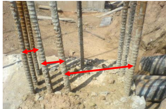
Column Steel Bars
