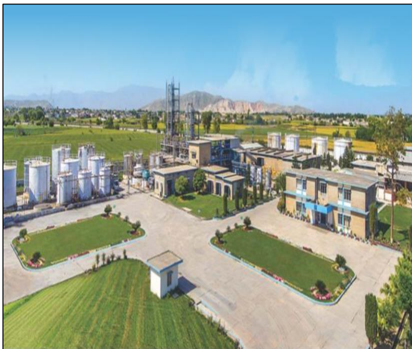
Figure 1.1 Wah Nobel Chemicals Plant
