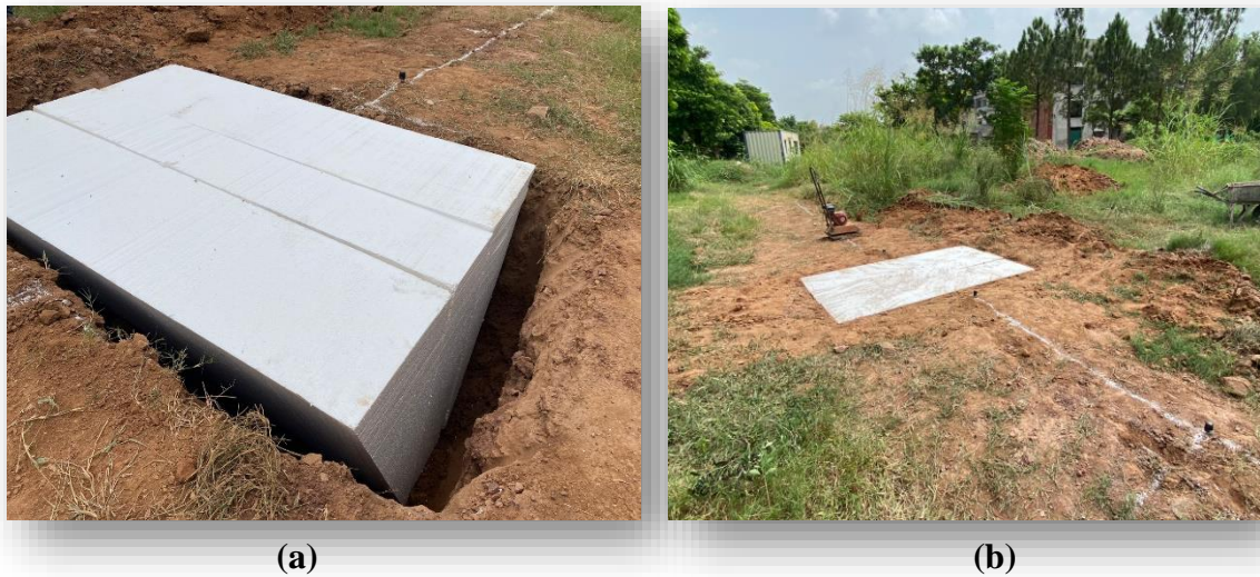
Figure 4.3: (a) EPS block placement (b) Eps filled trench measurements
