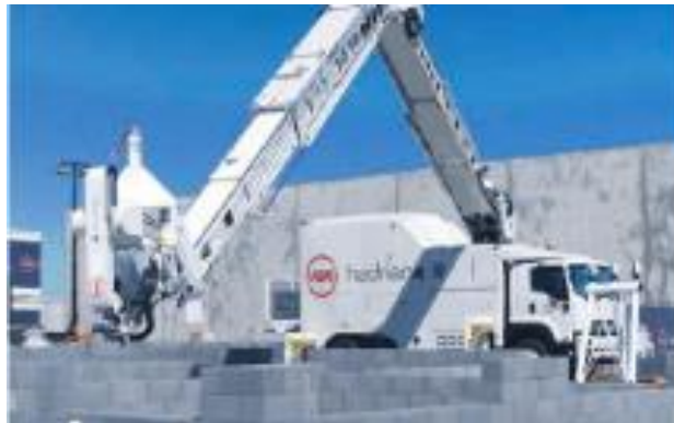
Figure 2.7: Hadrian X conveying concrete masonry units on a wall using its long telescopic boom (Melenbrink et al., 2020).
