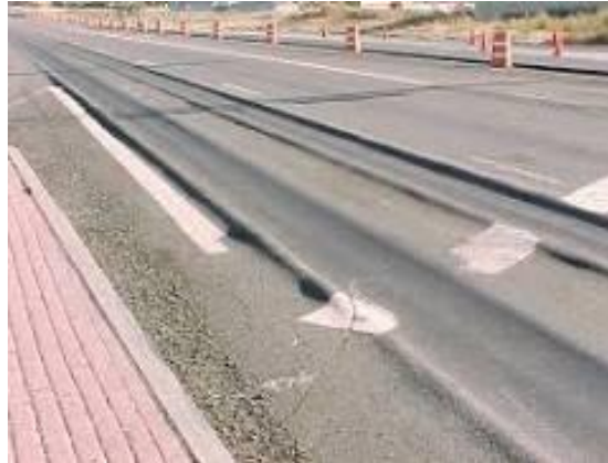
Figure 2.31 Pavement rutting
