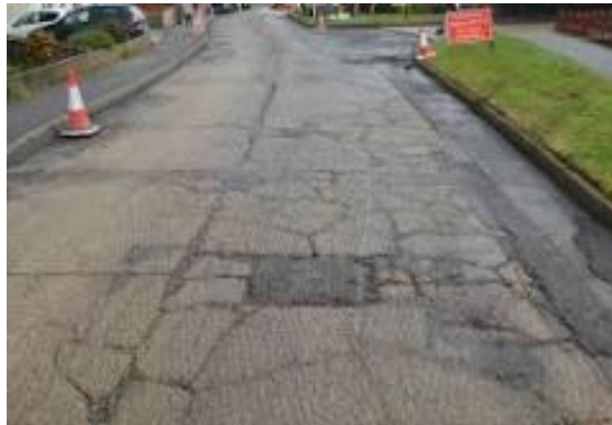
Figure 2.2 Pavement cracking
