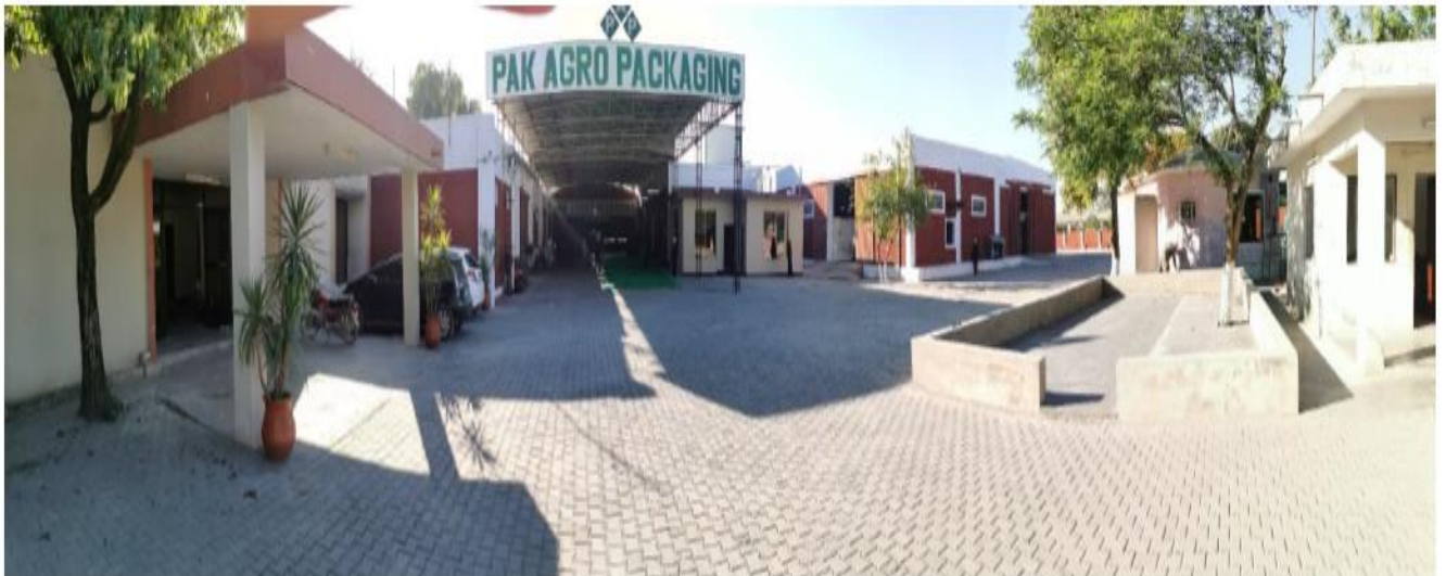
Figure 1.1.1: PAPL's Production Facility in Hattar Industrial Estate
