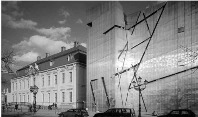
Figure 7 Image showing front Facade of the old and new building
