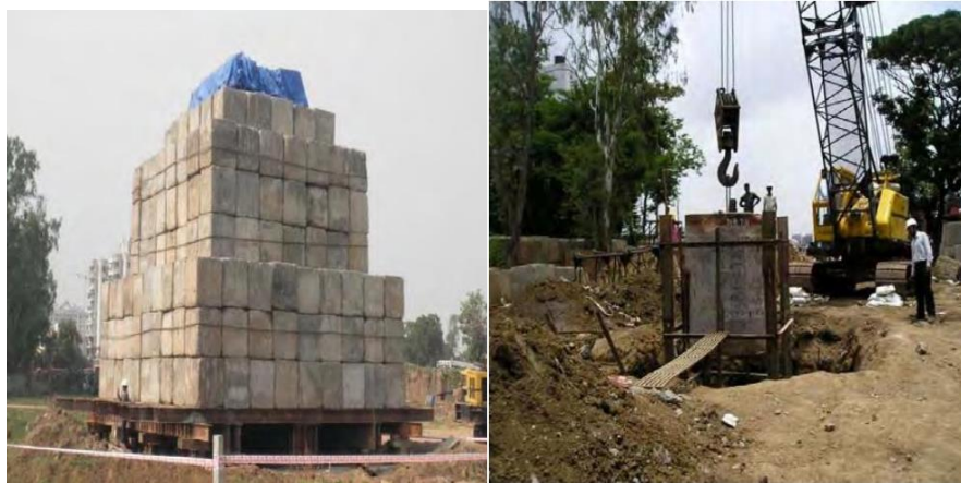
Figure 1.1: Dynamic load test and static load test at the site
