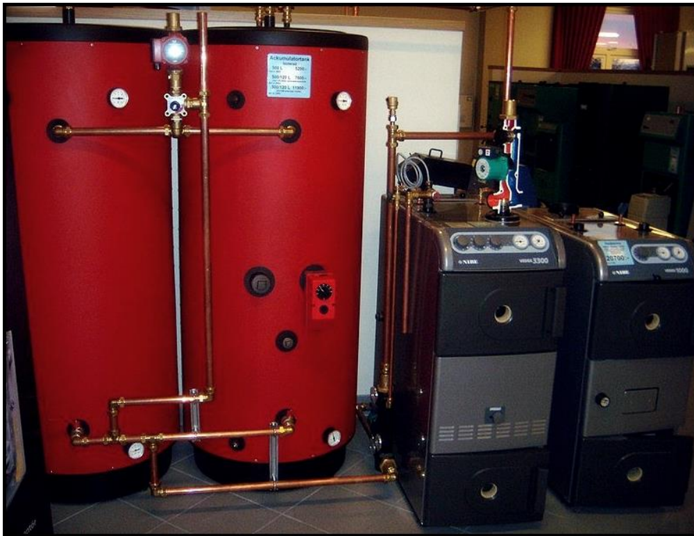
Fig 1.9) Hot water tank connected with furnace [15]
