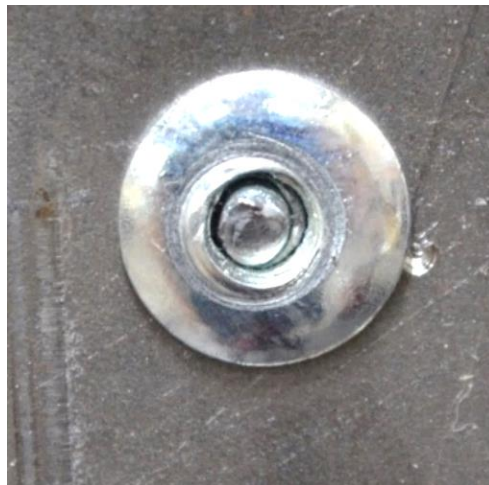
Figure 46 Installed rivet
