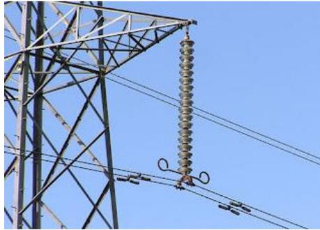
*Fig 1.2: Suspension insulator*
