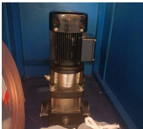
Figure 22: The 3-Phase Multistage pump
