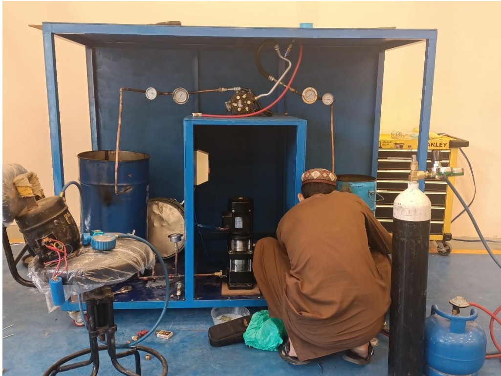
Figure 26: Careful Installation of Components
