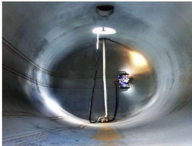
Figure 2: Remote inspection with robotic systems inspection by IRISNDT
