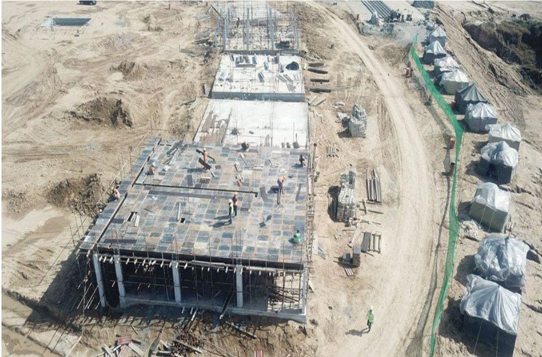
Figure 5 Eighteen Villas Construction site
